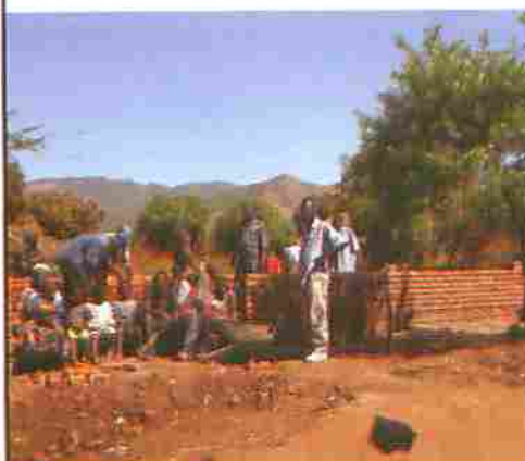
Work carries on with Bonzo's new house
